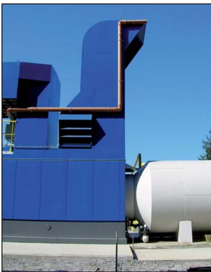
Fig.1 : G.T. with silencer
