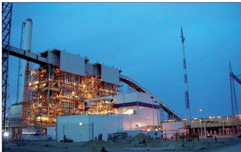
Fig.1 : General view of the TAMUIN plant (Mexico)
