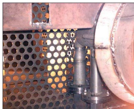
Fig.4 : Detail of the perforated grid located upstream the burners
