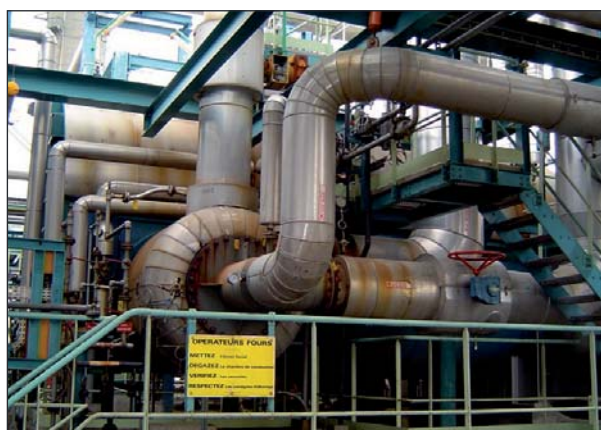
Fig.3 : Acid Gas burner - Front view
