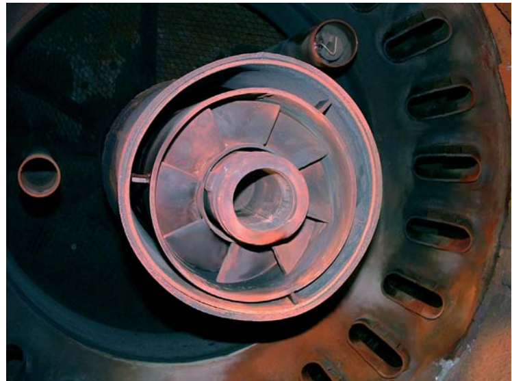
⇐ Fig.3 : Type K burner – EDF Richemont Power Station–400 MW boiler
