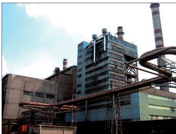
Fig.1 : Dunaújvaros Thermal Power Station
