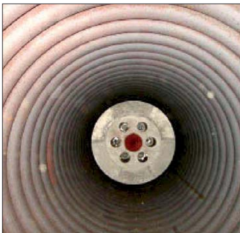
Fig.5 : Fire tube and burner view
