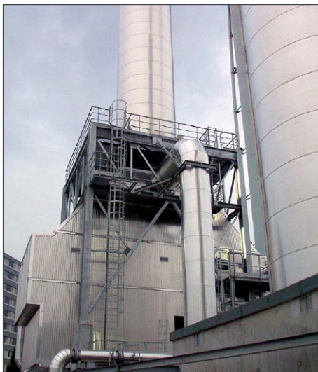
Fig.7 : FGR circuit connected to the stack
