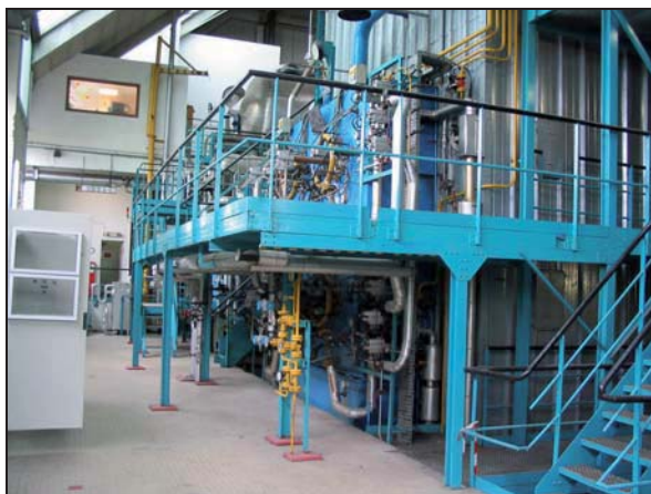
Fig.1 : Boiler n°2 before upgrading
