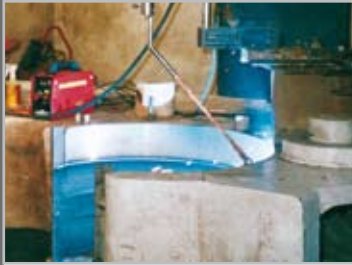
Mill being refurbished, resurfacing by automatic welding of a headstock
