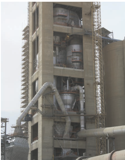
Fives FCB Low-NOx precalciner.
