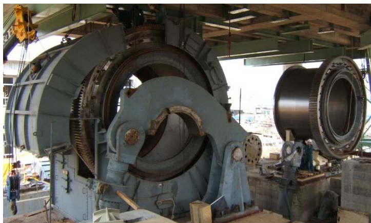
Figure 4: the mills during mechanical erection
